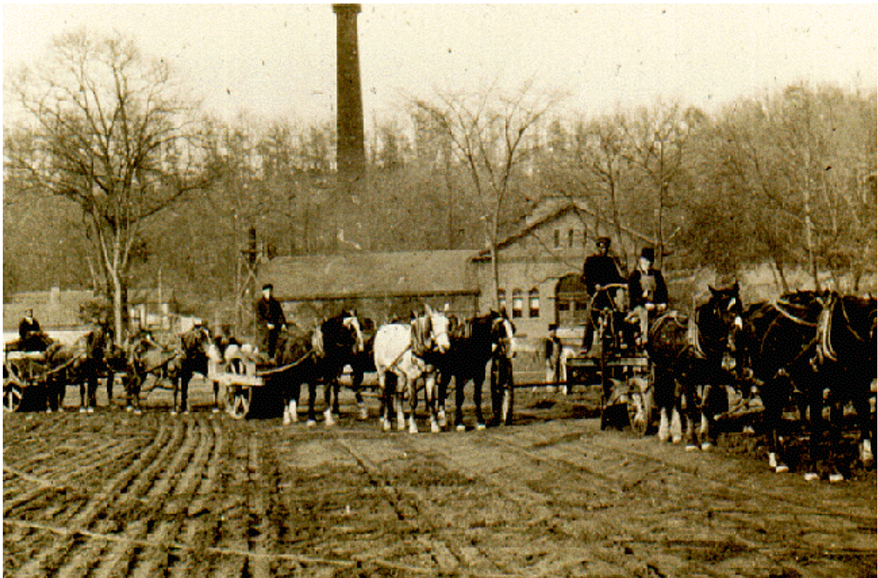
Horse-drawn Construction Equipment, Armory Street, 1902. These horse-drawn graders and roller are doing site preparation for the construction of the Whitneyville Slow Sand Filter. In the background is the then coal-fired Whitneyville Pumping Station with its 90 foot smoke-stack. To the left of the pumping station is one of the houses built by Eli Whitney in the 1790s as residences for workers in the Whitney Armory.
